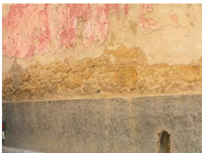
Lacuna no reboco
